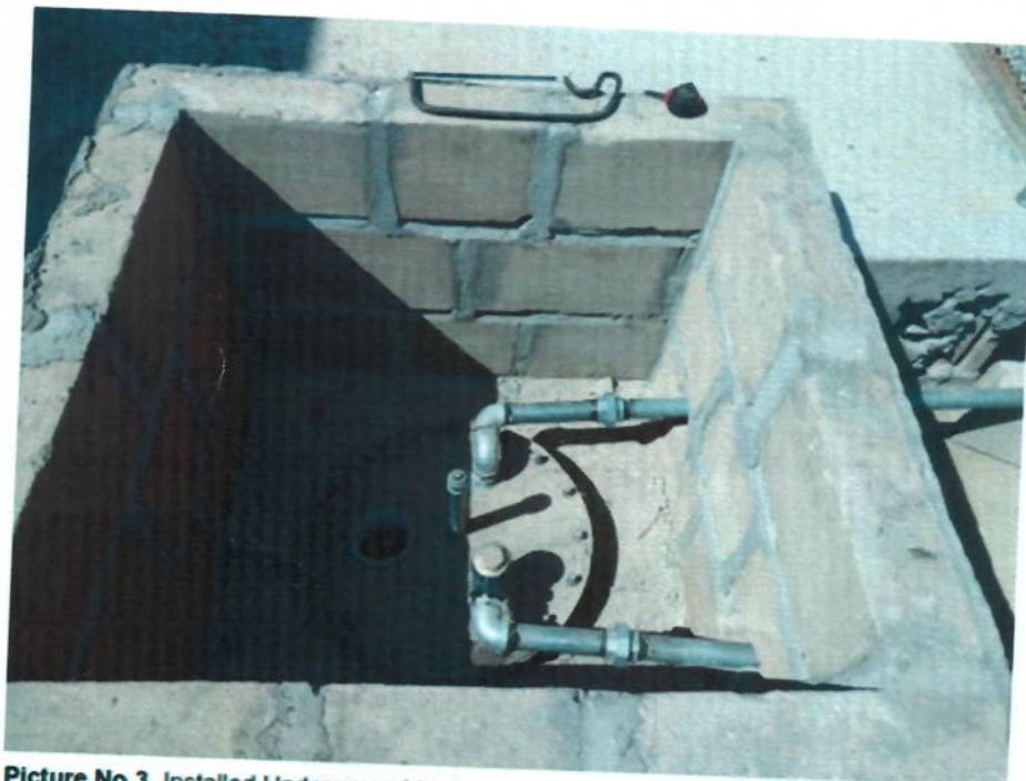
Picture No.3. Installed Underground tank
